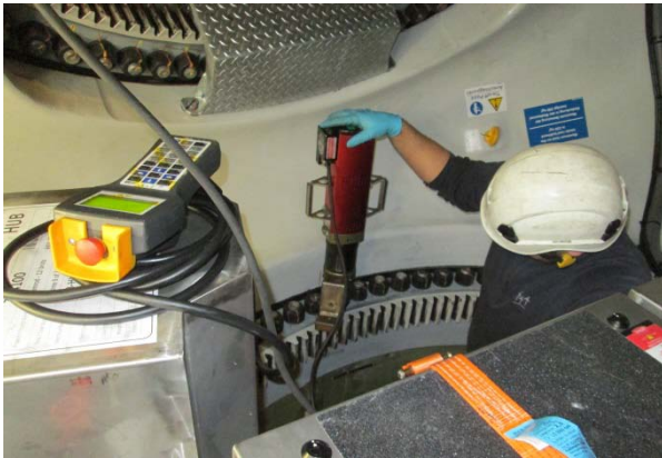
Figure 9: alkitronic® EF 300plus on a rotor blade
