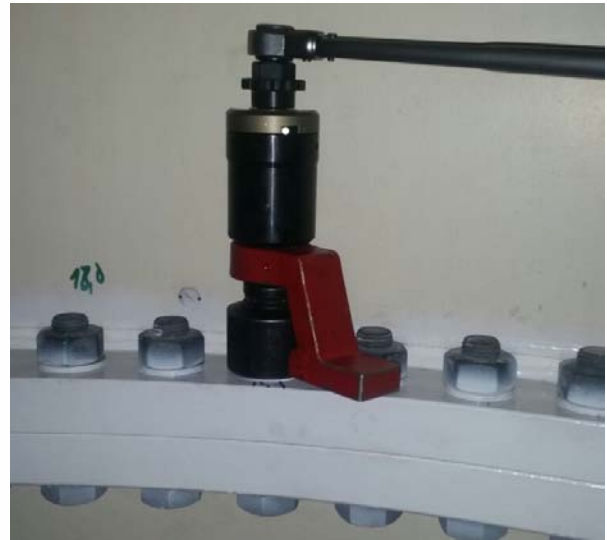
Figure 8: alkitronic® Manual torque multiplier HG 20 on tower bolts M36- high tension
