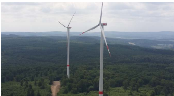
Figure 10: GE 2.8 on 140 m-hybrid tower
