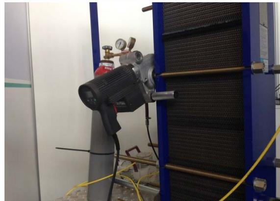
Figure 1: The alkitronic EFCip-R on a plate heat exchanger. Photo: alki TECHNIK
