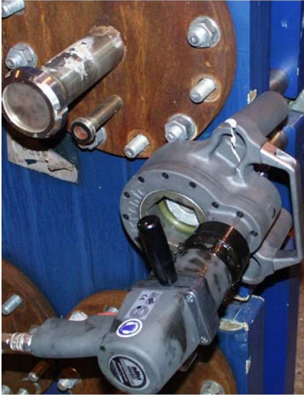
Figure 3: Bolting connection at the plate heat exchanger
